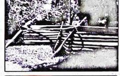
Asplit-rail fence is very simple to construct and can be assembled with few tools. They can even be disassembled if the fence needs to be moved or the wood becomes more useful for other purposes.
